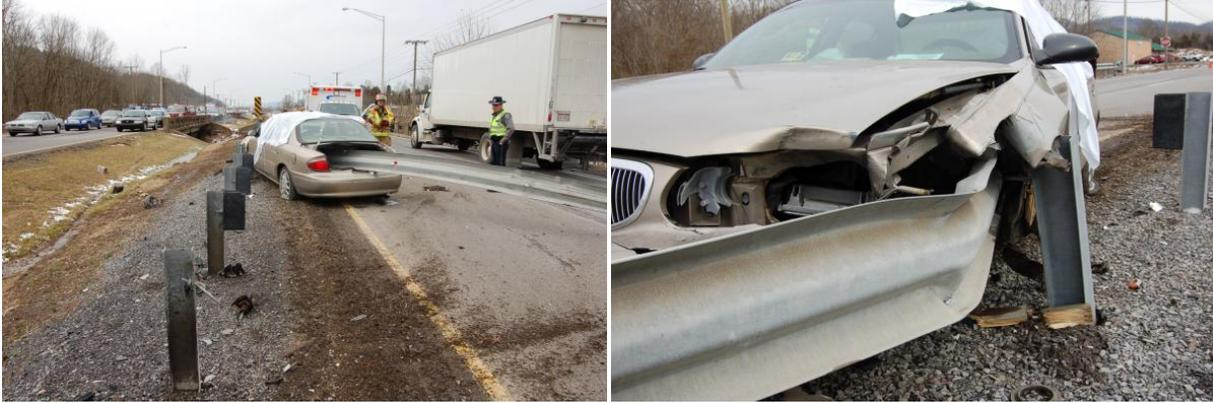
On the other hand, if the guardrail doubles over on itself after throat lock, it creates a new hazard for other approaching vehicles that may encounter the head before a maintenance crew can repair it. A doubled over guardrail after throat lock is shown below:
